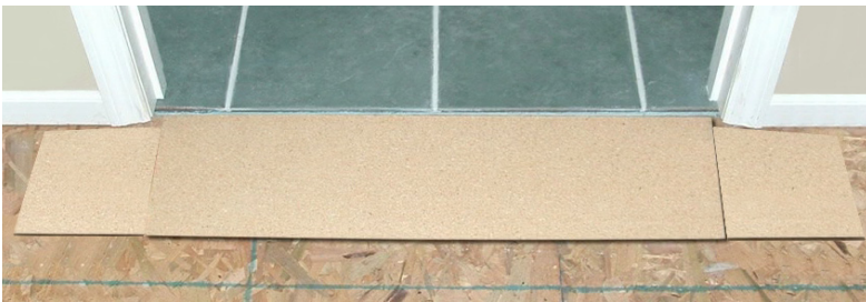
Ramp installed in 32" doorway with Composite Board Side Returns
