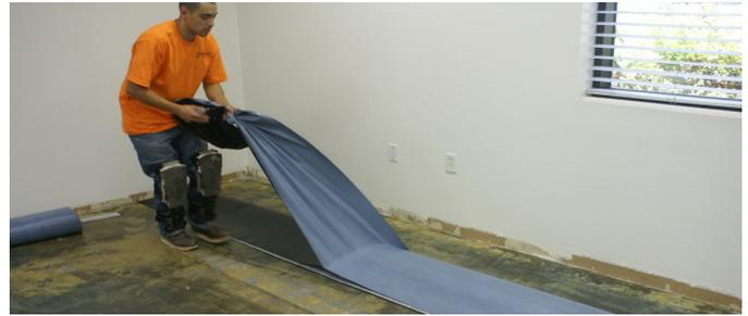
**STEP 2:** Fold back half the piece as illustrated. Continuously tear away the Release Liner at the midpoint perforation to expose the black adhesive. Then fold it back down and affix the TraxxShield99™ to the slab by pressing firmly with your hands. Allow the other half of the piece TO REST WITH THE LINER STILL ON.
