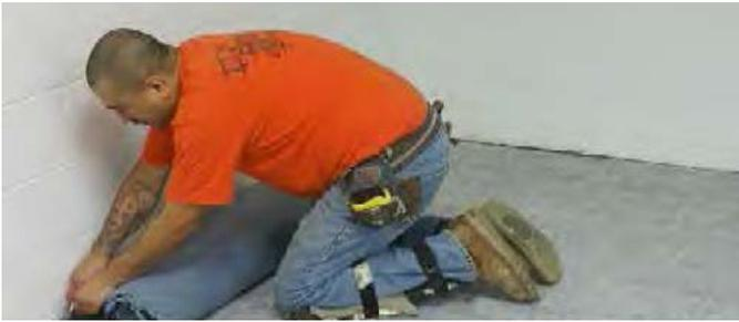
**STEP 1:** Starting at one corner of the room roll out TraxxShield99™ up to 1/8" from the wall and cut ends to the exact length using a utility knife. You may find that it is easier to handle a piece no greater than 15–20 feet in length.
