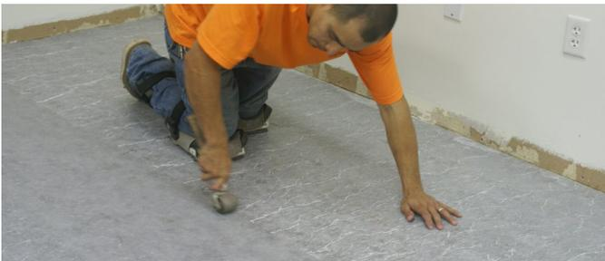
**STEP 7:** Then remove the Release Liner from one half of the second piece and press it down firmly as well. Be sure that the seam line is tight by using a hand roller.
