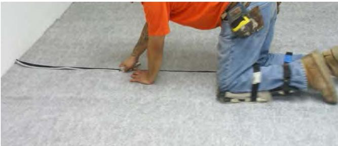
**STEP 3:** Proceed to line up the second piece of TraxxShield99™ and overlap the seam of the first piece by about 1-inch. Double-cut a new seam line through the overlapped pieces, and discard the cuttings. You have now created a tight seam line.
