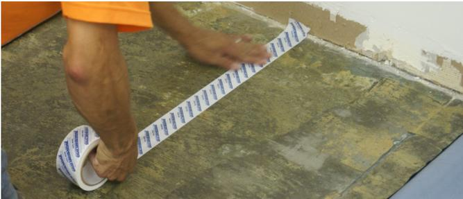
**STEP 5:** Then attach the tape to the slab and run along THE BOTTOM OF THE SEAM. Use a hand roller to ensure a good bond. The tape is specially formulated to support the moisture vapor suppression system, so it is imperative to use only TraxxShield99™ Seam Tape.
