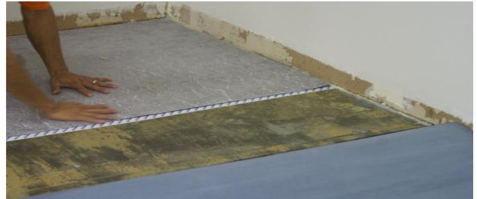
**STEP 6:** Proceed to remove the remaining Release Liner from the first piece and press down firmly over your tape line.
