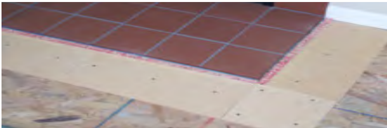
Composite Board Side Returns used to make an outside corner
